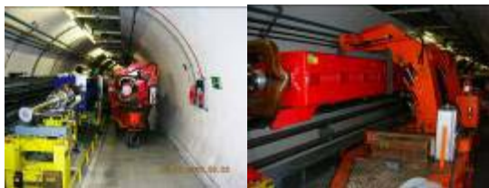
Figure 3: SPS magnet installation on the beam.
