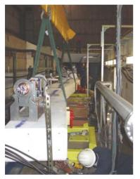
Figure 2: Installing the girder supporting the BPM3-5 triplet.
