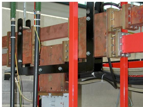
Fig. 2: R32 variable power divider consisting of three 3dB coupler and two sliding shorts (lower part).
