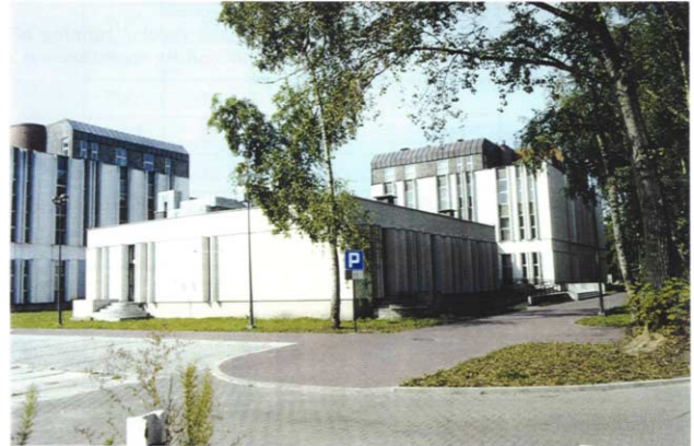
Fig 1. Heavy Ion Laboratory building
