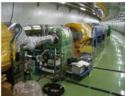
Figure 2: Magnets and beam duct in the MR ring tunnel. The vacuum evacuation test is in progress.
