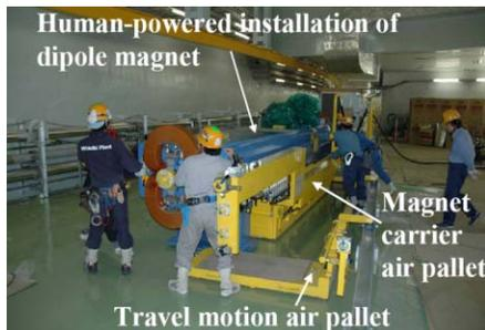
Figure 2: air float transportation system
