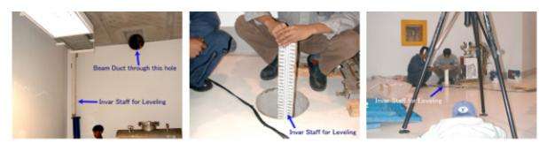
Fig.10 The Invar Staff comes through the floor hole from the downstairs in order to connect to the height between downstairs and upstairs.
