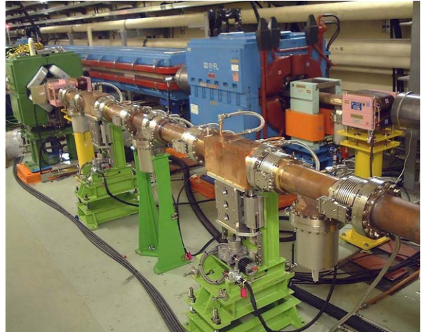
Fig. 4 Movable mask installed in the tunnel.
