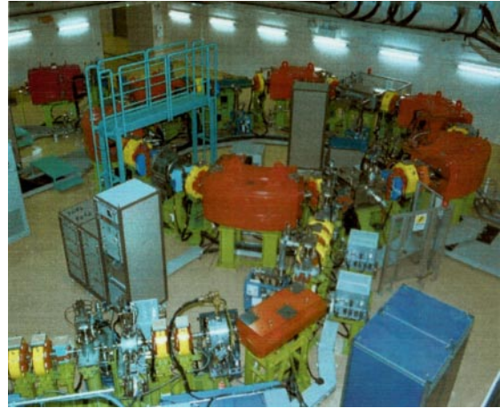
Fig. 9: A 250 MeV synchrotron ring at University of Tsukuba. An injection line can be seen on this side and an extraction line is on the other side.
