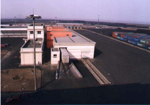
Figure 11: building and working field for the inspection system at the Tianjin seaport customs
