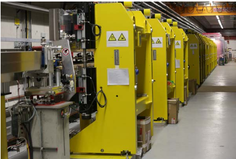
FLASH2 variable gap undulators
