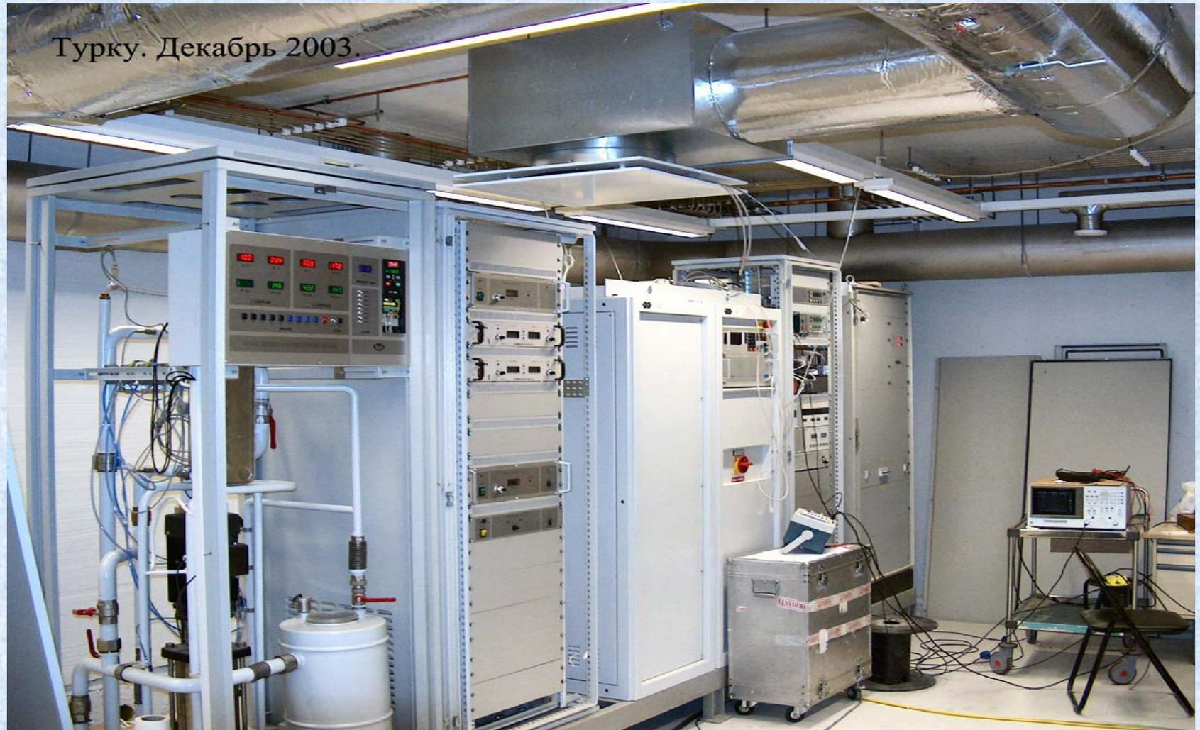
The distributed automated control system is built on the basis of programmable logic controllers PLC produced by the Mitsubishi firm. The PROHIBUS and ETHERNET interfaces for data transmission are used.
