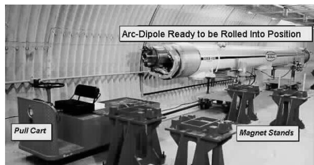
**Figure 3: Dipole Installation**
