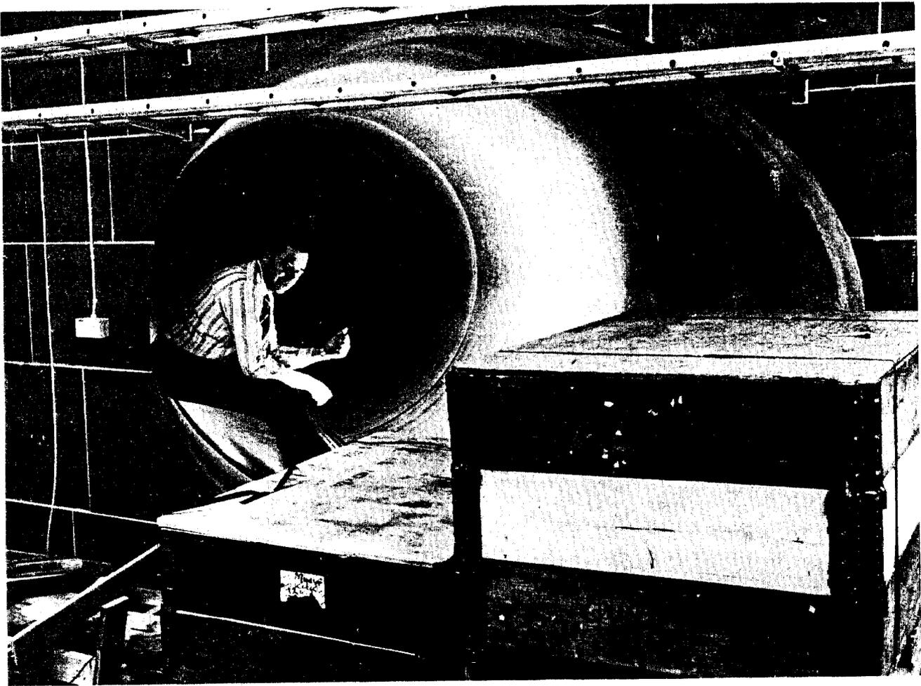
Fig.3. Matchboxing P.M. Author pointing into the 8 m deep beam-dump tunnel (B) (cf figs. 1 and 2). This is the most probable site for the first radionuclide-producing beam-dump. Left-over protons from the production of neutrons for (n,p)-experiments will be directed into the tunnel by two bending magnets and focussed on the beam dump by a quadrupole. (Photo. T Thörnlund. Reproduced with permission from the GWI Info-Dept.)
