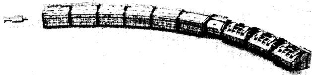
Fig. 3 The superconducting extraction channel before welding into its liquid helium container. (The "strongback" on which the modules are mounted is 80 mm high.)
