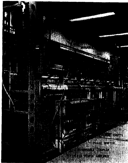
Fig. 9. L/2 loop installation (downstream view).
