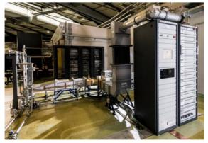
Figure 5: SSPA transmitter for the ALBA booster.
