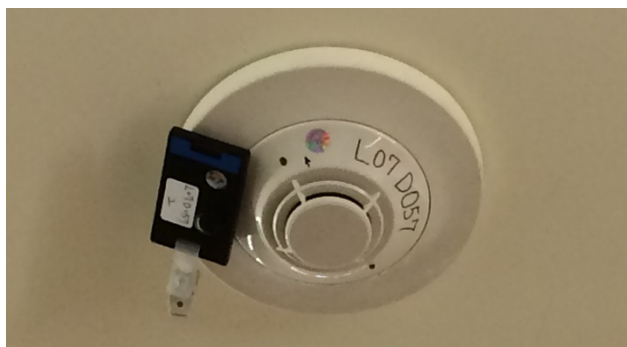
Figure 5: Detector installed in the TPS tunnel with a TLD.
