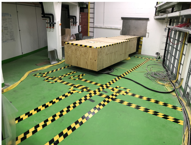
Figure 4: Detailed view on the granite block. The hole to the X-ray hutch is closed with a 25 cm thick lead shielding. Tape on the floor illustrates the path of the laser beam lines to the test area and the granite block, to be installed mid 2019. Also these elements will be located under a false floor.
