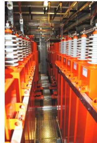
Replacement of main dipole power converter (for 10 T/s, 50 MW)
