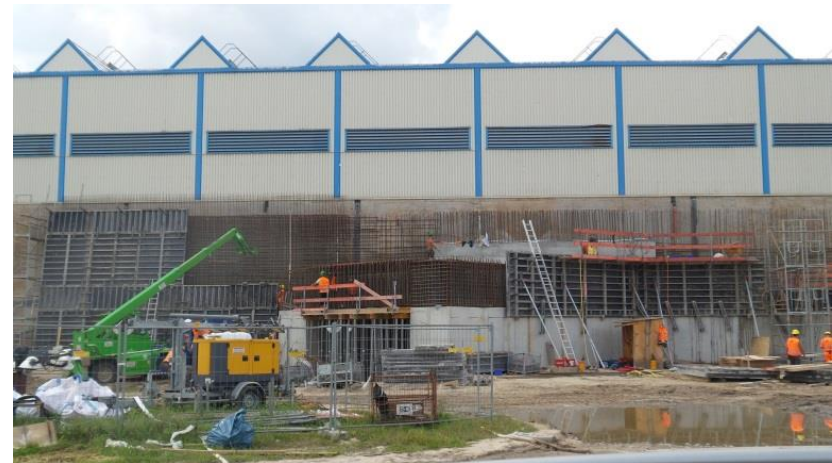
Interface for FAIR tunnel 101 completed.
