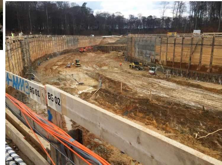
Excavation of SIS100 tunnel. Present depth: -16 m
