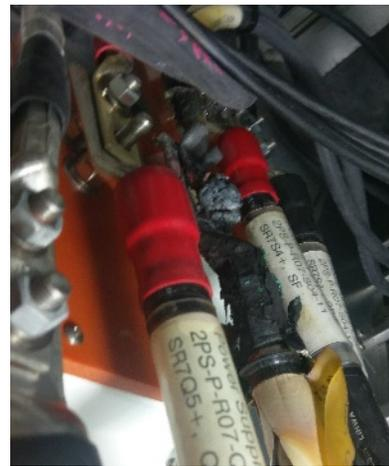
Figure 7: The burn out of the cable terminal of QS5-0705 causing spikes.
