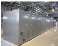
Figure 7: New dipole magnet PS in D4.
