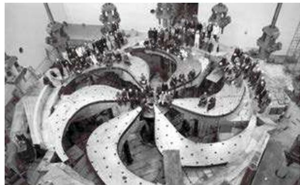
Figure 1: Staff on the lower magnet (Jan 1972). Note the single aluminum coil (with V-shaped connectors) and the studs along each magnet edge for the steel shim plates.
