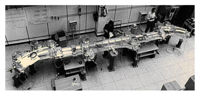
Figure 1: One of the arcs of the DA $\Phi$ NE positron ring, under testing at the LNF vacuum laboratory.
