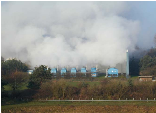
Figure 1: The HERA wet cooling towers on a day with more than 95% relative air humidity
