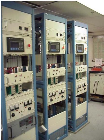
Figure 2: Charging Power Supply Racks picture
