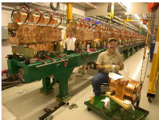
Figure 7: CCL bridge coupler installation preparation.
