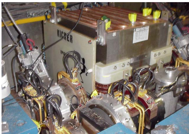
Figure 4: The IPF kicker magnet as installed in the LANSCE transition region. Upstream end of the magnet is to the left.
