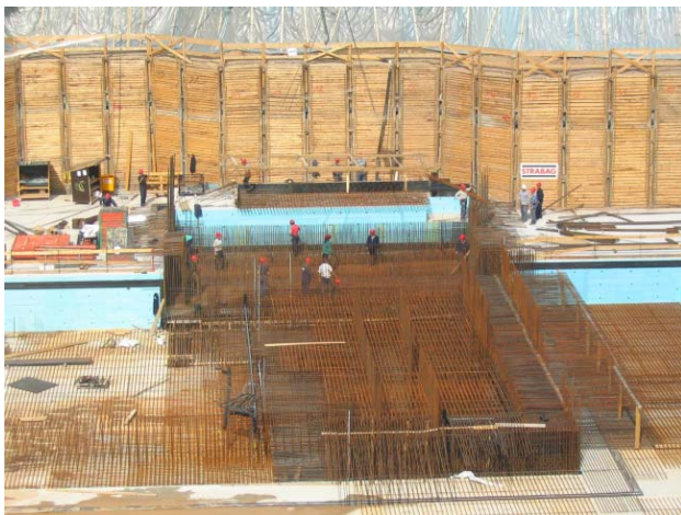
Figure 3: Preparation work for the gantry floor (06/04)
