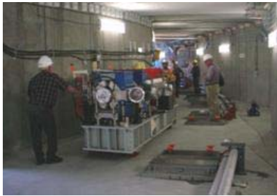
Figure 3: Installation of magnet rafts on new floor in tunnel.
