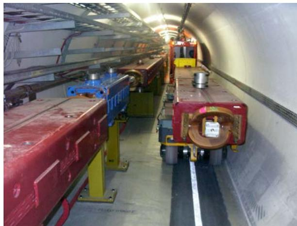
Figure 2: TI 8 during magnet installation
