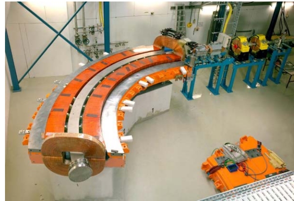
Figure 6: Gantry segment (the upper yoke of the 90° dipole and its mirror plates not yet installed).
