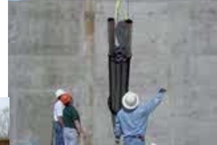
Installing transferline
