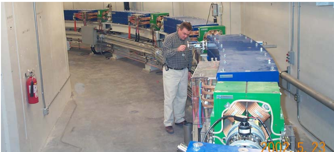
Figure 5: Fully installed section of the booster synchrotron with 4 girder.
