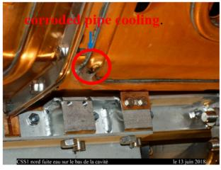
Figure 4: Corroded Pipe Cooling.
