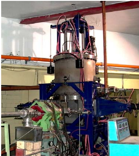
Fig. 1. Photograph of the new Rebuncher
