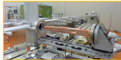
Figure 4: Installation fixtures for crotch absorber installation.
