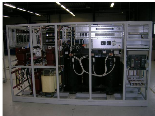
Figure 2: Picture of the dipole PC.
