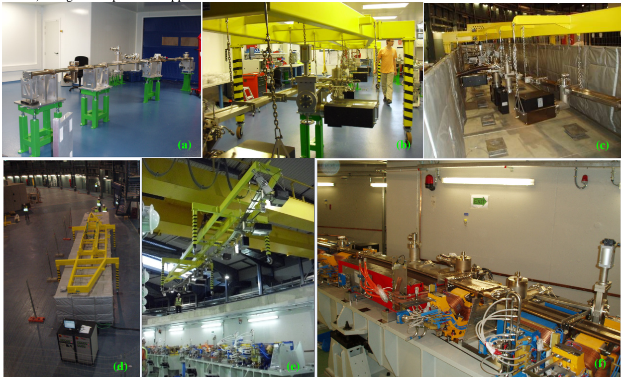
Figure 3: the installation of the storage ring sectors: a) preassembly and testing in the clean room, b) connection of the strong back, c) the sector inside the bakeout oven, d) bakeout to 200°C inside the oven, e) moving the sector after the bakeout under vacuum into the tunnel with the magnets open, f) placing the sector on the supports on the girder.
