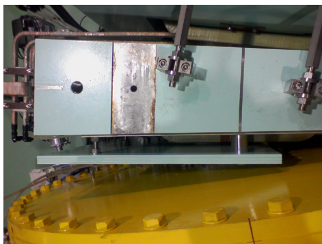
Figure 7: Installed additional field clamp at cavity section.
