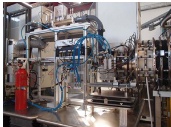
Figure 1: Layout of ISHP source: the klystron, the RF chain and components, and the plasma chamber are installed on a high voltage platform.
