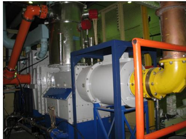
Figure 3: RF generator with part of a feeder (to the right).
