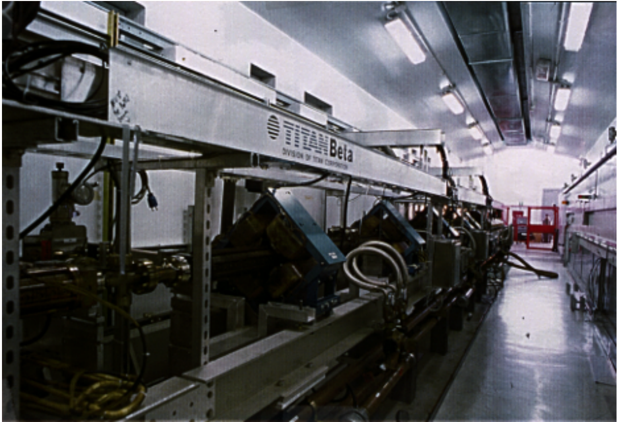
Figure 2: DAΦNE LINAC during installation (April 95).
