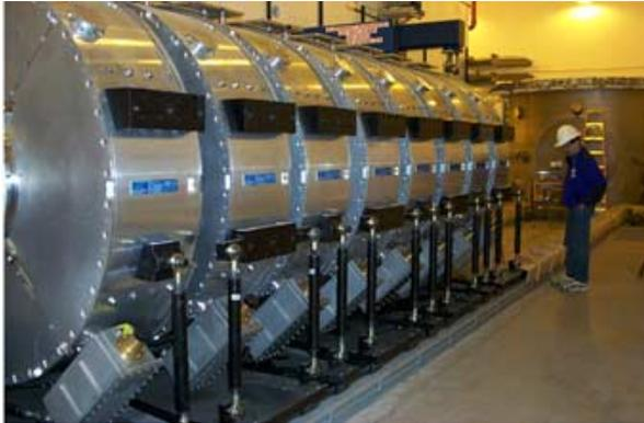
Fig. 6 The large bore induction cells during installation immediately downstream of the injector
