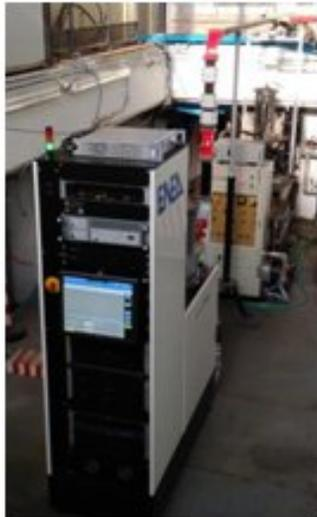
Figure 6: (Left) Scandinova K1 Modulator + TH2157A klystron installed on TOP-IMPLART accelerator.
