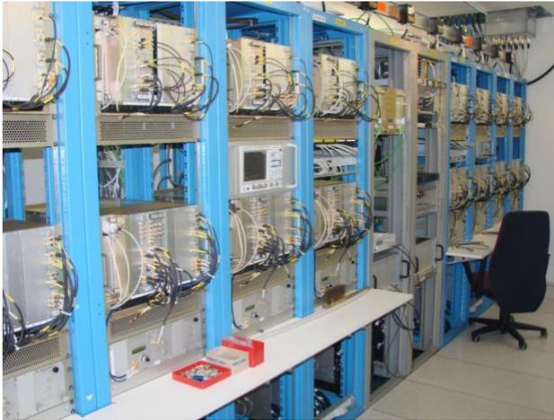
Figure 4: Cavity Controllers in UX45 Faraday Cages.
