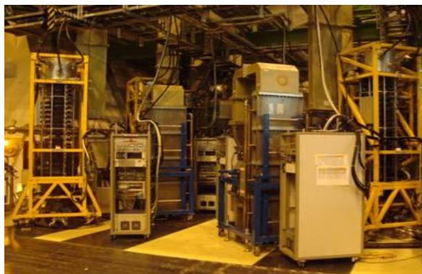
Figure 2: Klystrons, Power Equipment and Control Racks in the UX45 Cavern.
