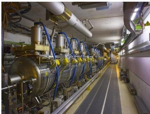
Figure 1: RF Cryo-modules in the LHC tunnel at IP4.
