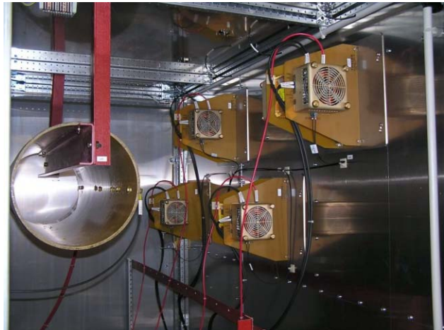
Figure 4: Filament and Grid Power Supplies
