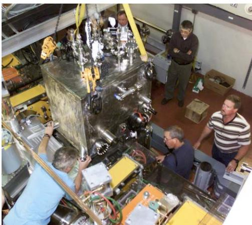
Figure 2: Installation of the first Superbend.
