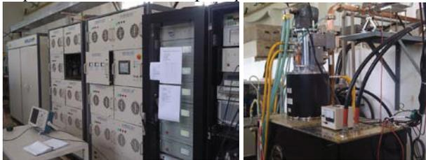
Figure 9: The modulator and Toshiba E37311 klystron.
